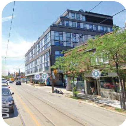
Dundas Street West and Sheridan Avenue
